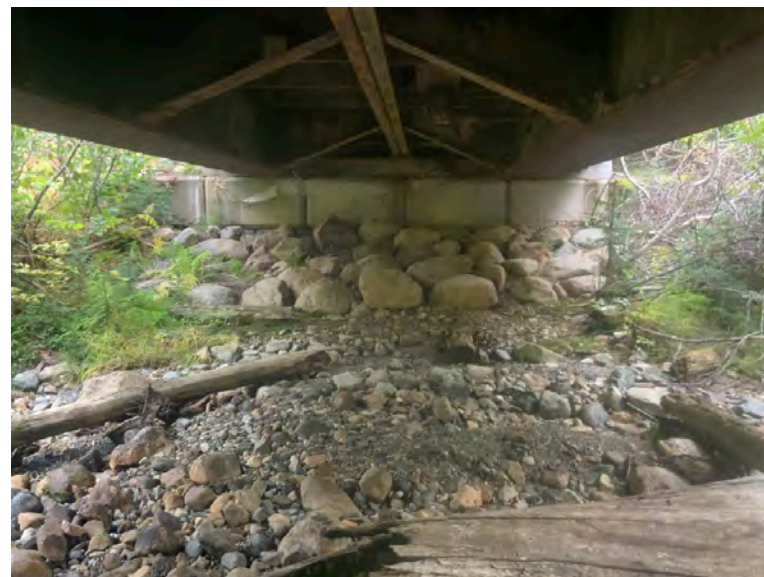
Right Bank Abutment when facing downstream
