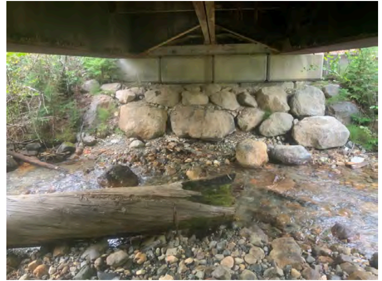
Left Bank Abutment when facing downstream
