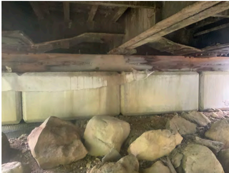
Right Bank Abutment when facing downstream
